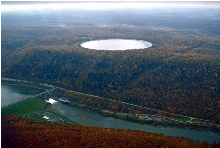
Seneca pumped storage and hydroelectric facility, Warren County, Pennsylvania
